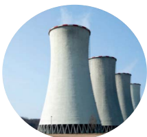
Cooling & Process water disinfection
