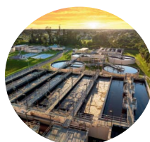
Industrial water treatment
